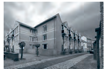
21 residential buildings on the Gasthuisstraat, Grave (1975).
